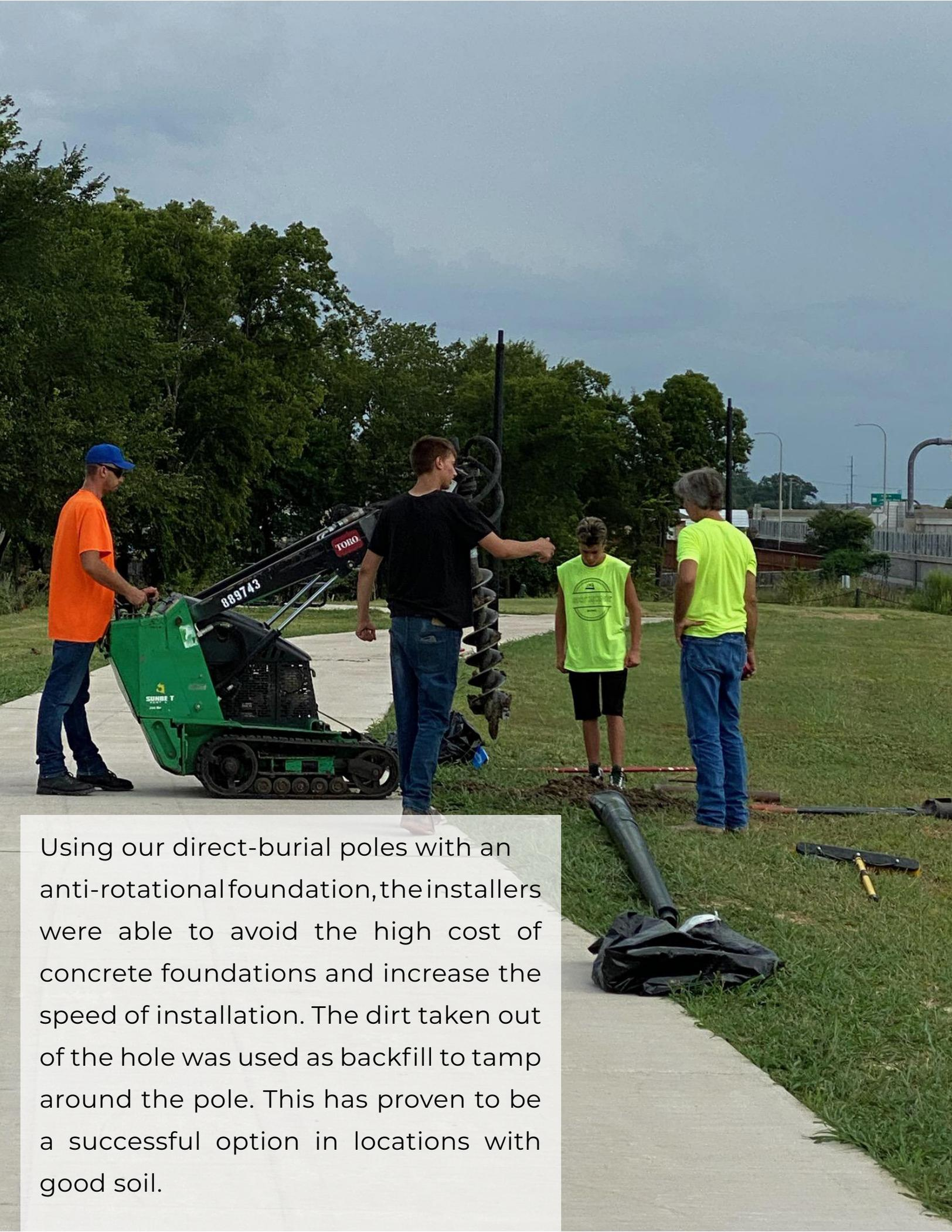
Using our direct-burial poles with an anti-rotational foundation, the installers were able to avoid the high cost of concrete foundations and increase the speed of installation. The dirt taken out of the hole was used as backfill to tamp around the pole. This has proven to be a successful option in locations with good soil.
