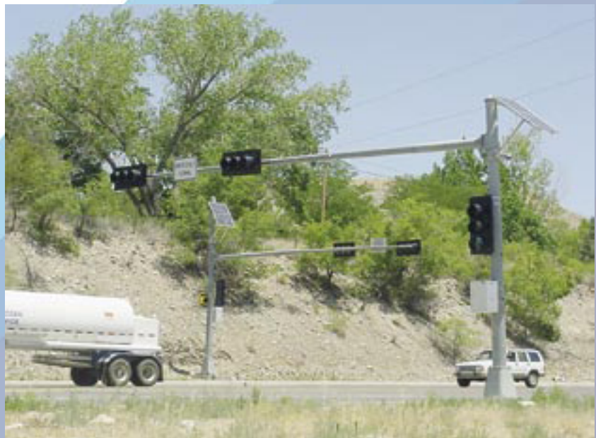
Three 3-section signal heads (solar powered). Lights are green until fire station activates.
